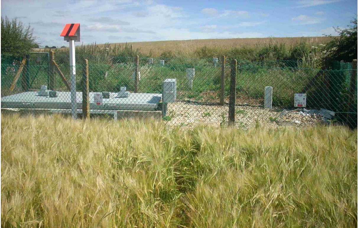
Figure 3.6 Photograph of an existing valve enclosure and flight marker post
